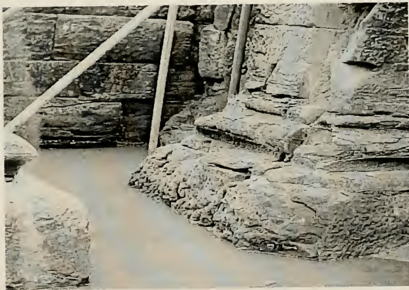
Figure 1.5: Unsheltered room retains water on the floor for several days before the water evaporates. The Northern Gopura of the Phimai Sanctuary, June 2000
