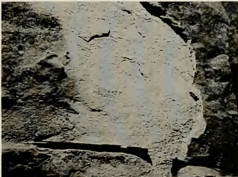
Figure 4.2: Scaling of sandstone surface The deeper dampness in the stone leads to the flaking and scaling of the stone surface. The condition of the stone wall of the Northern Gopura. (June 2000)
