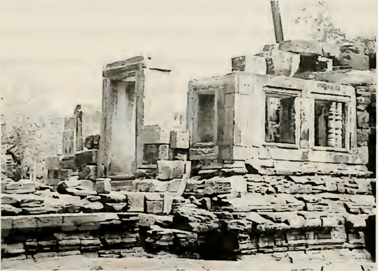
Figure 1.12: New stone replacement during anastolysis restoration project. (Fine Arts Division, the Department of Interior, 1998)
