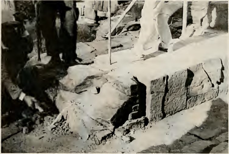
Figure 1.11: Ancient stone block broke during the restoration project. (Fine Arts Division, the Department of Interior, 1998)
