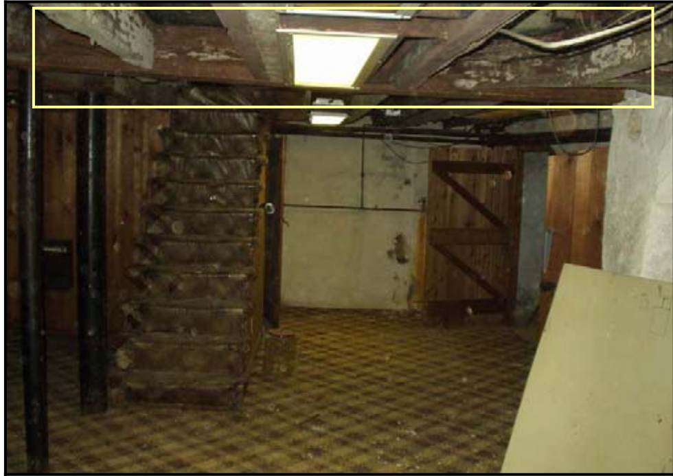
Figure 14: Deflected steel beam in basement (Photo 2004)
