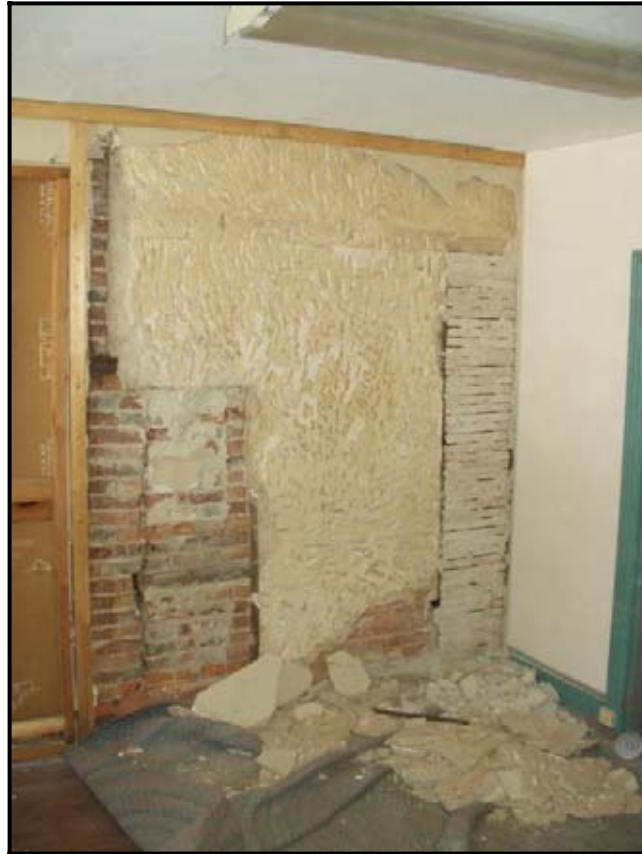
Figure 36: Damaged 19 th century plaster on east wall of Room 1-5 (Photo 2004)
