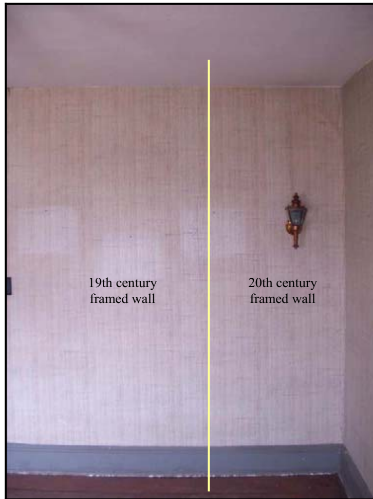
Figure 24: Seam on west wall of Room 1-1. Evidence of original framed wall section (Photo 2004)
