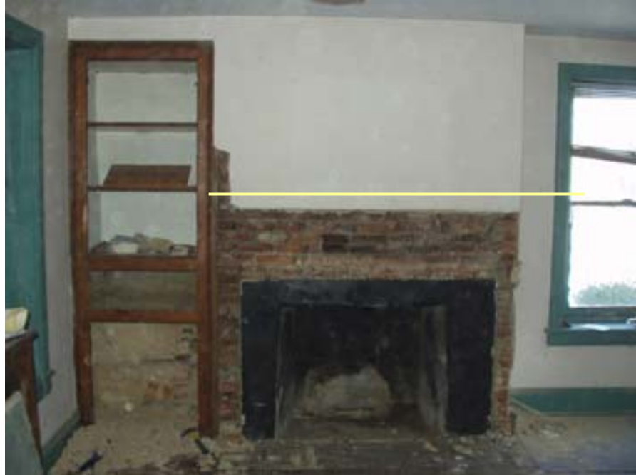
Figure 33: Seam in plaster above fireplace in Room 1-5 (Photo 2004)
