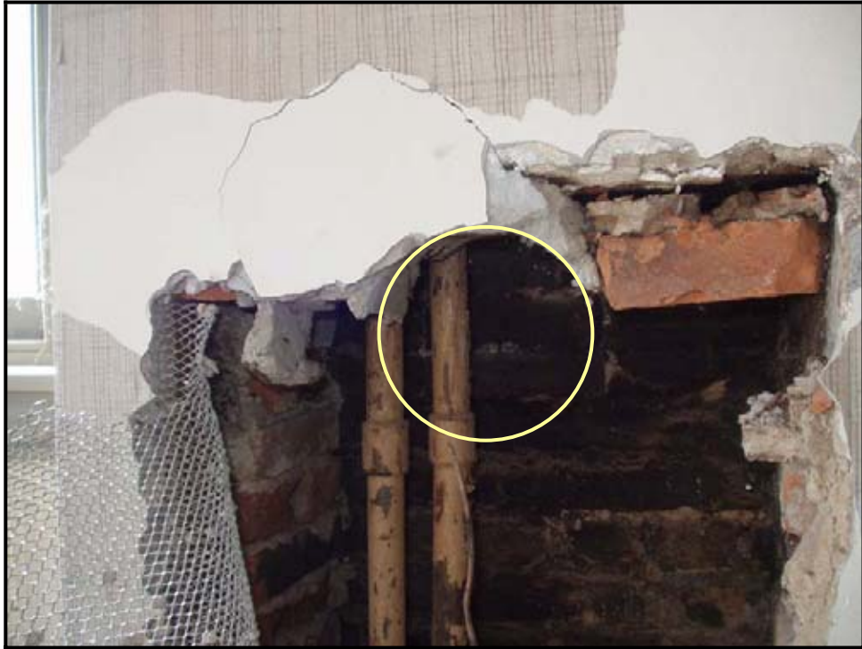
Figure 23: Evidence of a stove pipe in fireplace system in Room 1-1 (Photo 2004)
