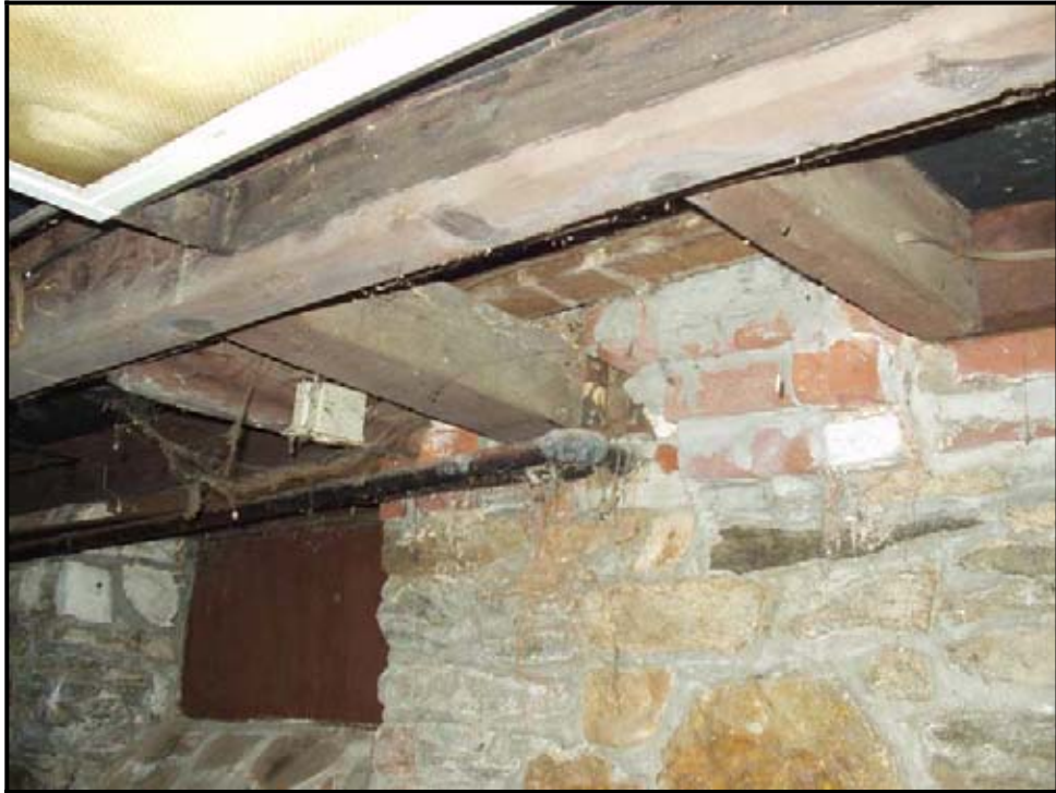
Figure 15: Replacement fireplace support at southern end of basement (Photo 2004)
