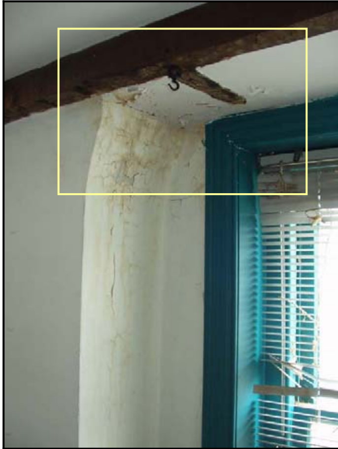
Figure 39: Chimney system in Room 2-6 shortened (Photo 2004)
