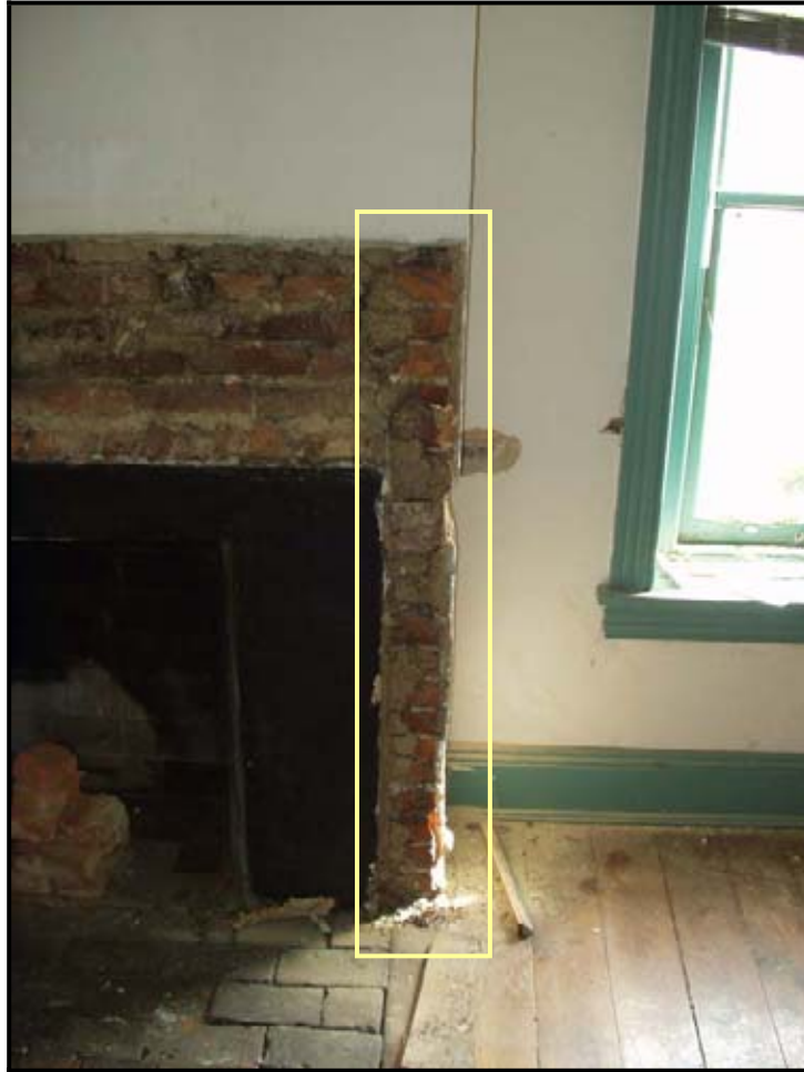
Figure 31: Evidence of a cheek wall for a large cooking fireplace in Room 1-5 (Photo 2004)
