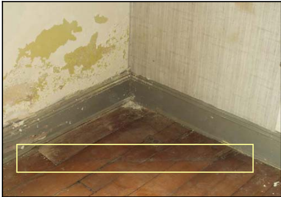
Figure 20: Worn mark in southeastern corner of Room 1-1 indicative of corner cabinetry (Photo 2004)
