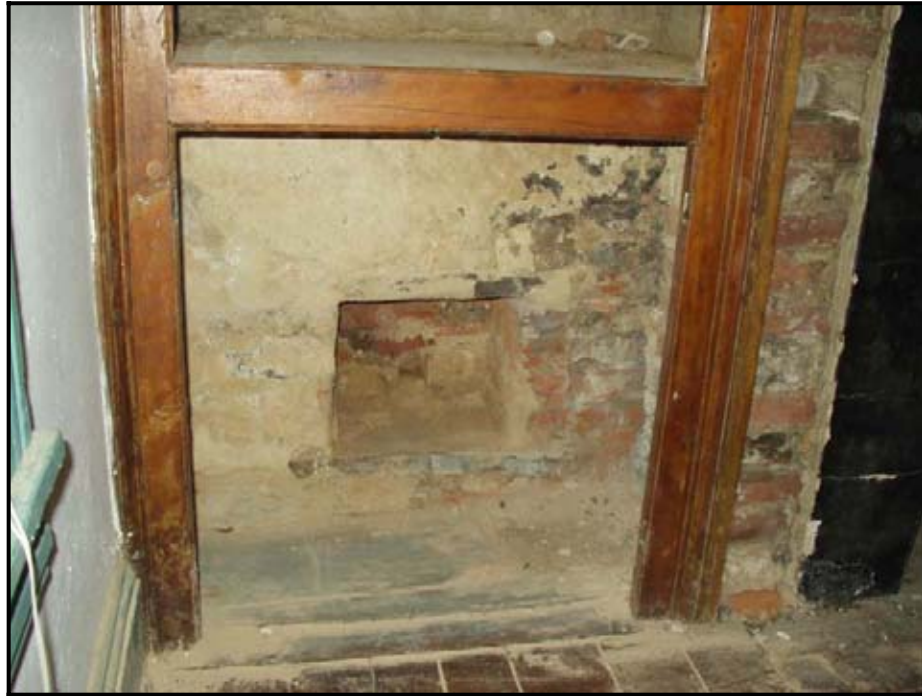
Figure 34: Stone lintel and niche on west side of fireplace in Room 1-5. Evidence of a bake oven. (Photo 2004)
