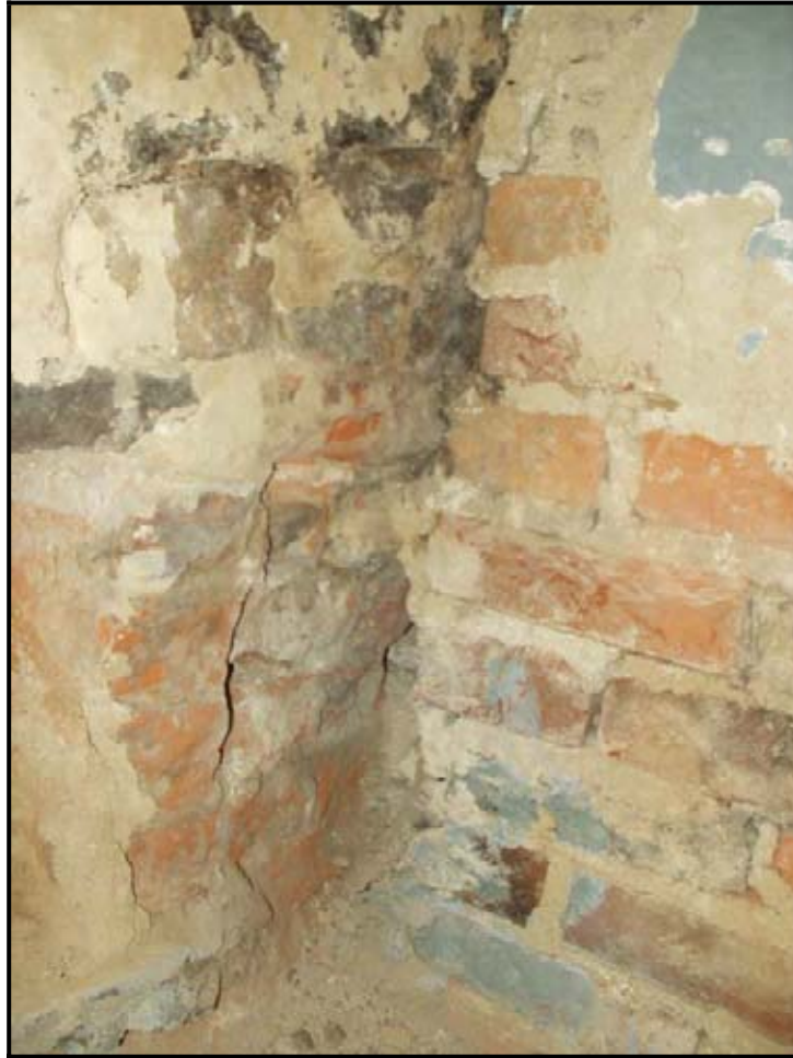
Figure 32: Brick on west side of fireplace not keyed in to exterior masonry in Room 1-5 (Photo 2004)
