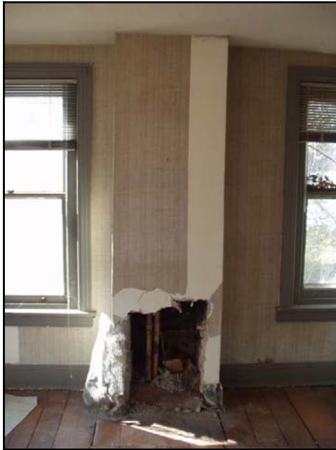
Figure 22: Closed fireplace system in Room 1-1 (Photo 2004)
