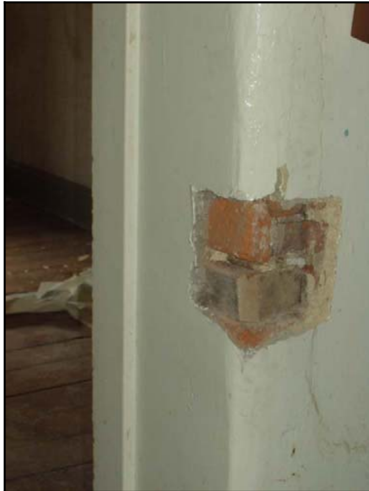
Figure 27: Wood nailing block on west wall of Room 1-2 (Photo 2004)
