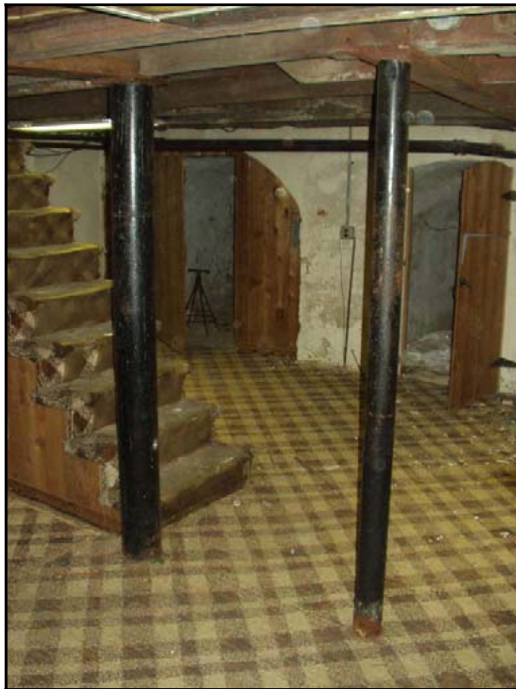
Figure 13: Steel columns supporting summer beams in basement (Photo 2004)
