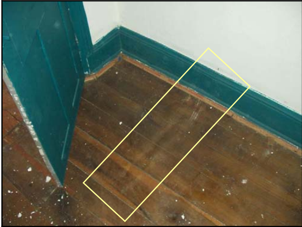
Figure 41: Shadow on floor of Room 2-6, evidence of a framed wall (Photo 2004)
