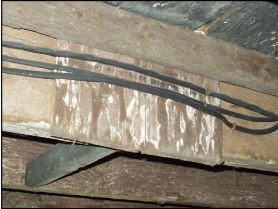
Figure 16: Remnants of partition boards within framed staircase opening in basement (Photo 2004)
