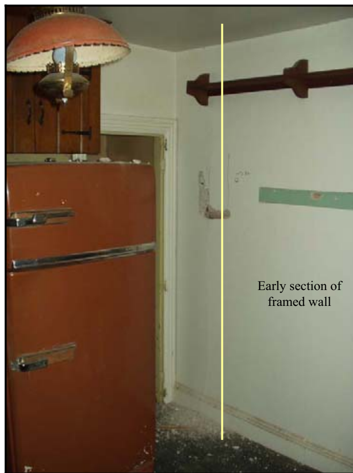
Figure 25: Seam on east wall of Room 1-2. Evidence of original framed wall section (Photo 2004)
