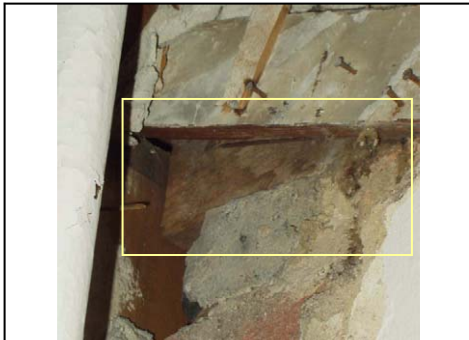
Figure 37: Remnants of a wooden lintel adjacent to window on west wall of Room 1-5 (Photo 2004)
