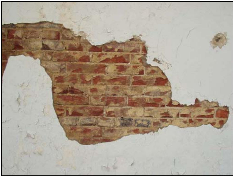
Figure 11: Damaged brick underneath stucco on west facade (Photo 2004)
