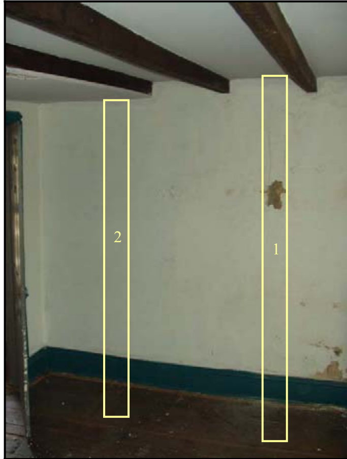
Figure 40: Seams on west wall of Room 2-6, indicative of two different walls (Photo 2004)
