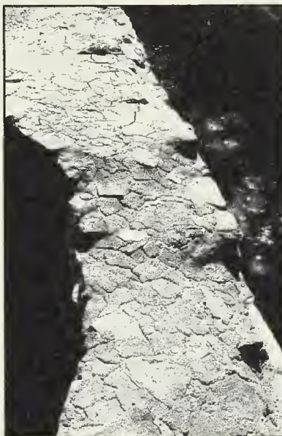
Figure 7. Cracking of acrylic emulsion-modified soil capping is a problem experienced at Aztec Ruins National Monument. But the cracks are a function of the mineral components of the soil mix, particularly the clay minerals, and not the acrylic amendment. The cracks are a cause for concern because they allow more water to enter the interior spaces of the walls.
