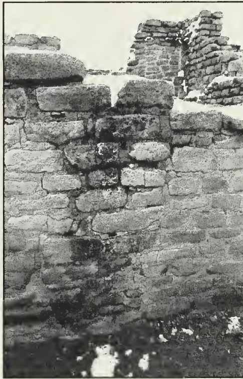
Figure 8. Water in the form of melting snow is one of the deterioration mechanisms at work on soil mortars in the Southwest. This photograph of Far View Ruin at Mesa Verde National Park reveals the wet stain of water flowing over the wall face after a fall snow. The wall is not wetted equally, and some areas are wet more often, and remain wet longer, leading to soil mortar erosion. (See Appendix A for SEM views of sound and deteriorated mortar from this ruins site.)
