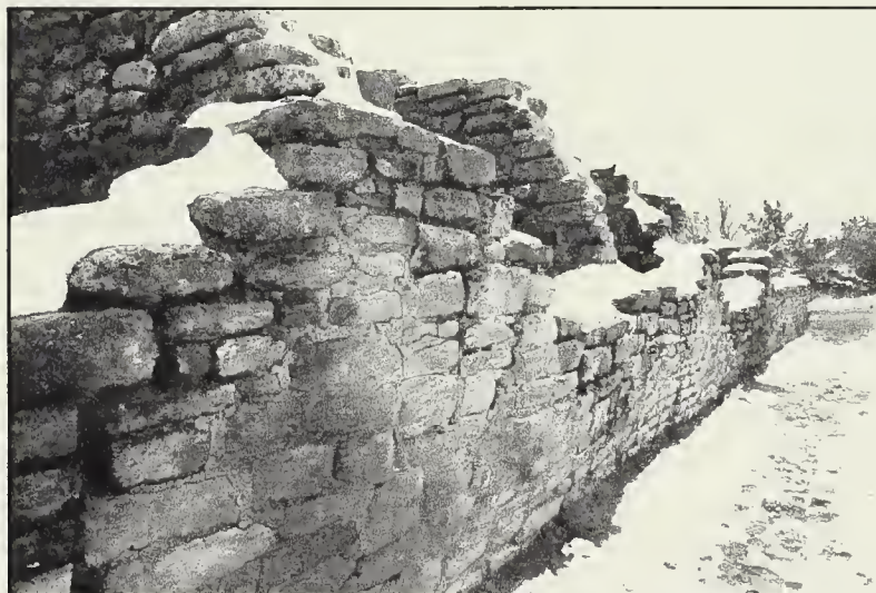
Figure 20. The climate of the Colorado Plateau, with year-round rain and snow, and broad temperature fluctuations, places great stress on the earthen components of remaining Anasazi architecture. The challenge of maintaining the ruins while using visually and physically sympathetic materials is great.
