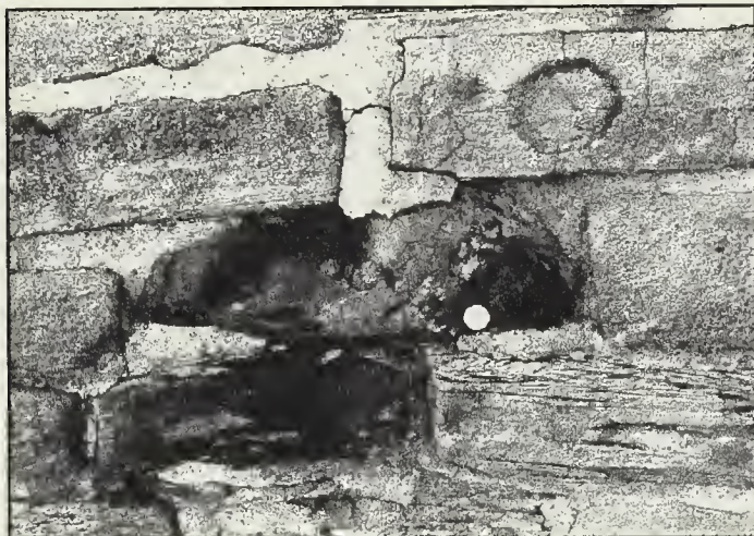
Figure 2. These sandstone masonry blocks at Aztec Ruins National Monument are eroding at a faster than normal rate because of the adjacent Portland cement-based mortar. The deleterious effects of cementitious mortars are one reason the National Park Service has shifted to more compatible acrylic emulsion-based earthen mortars at some ruins sites in the Southwest. (A quarter is shown for scale.)
