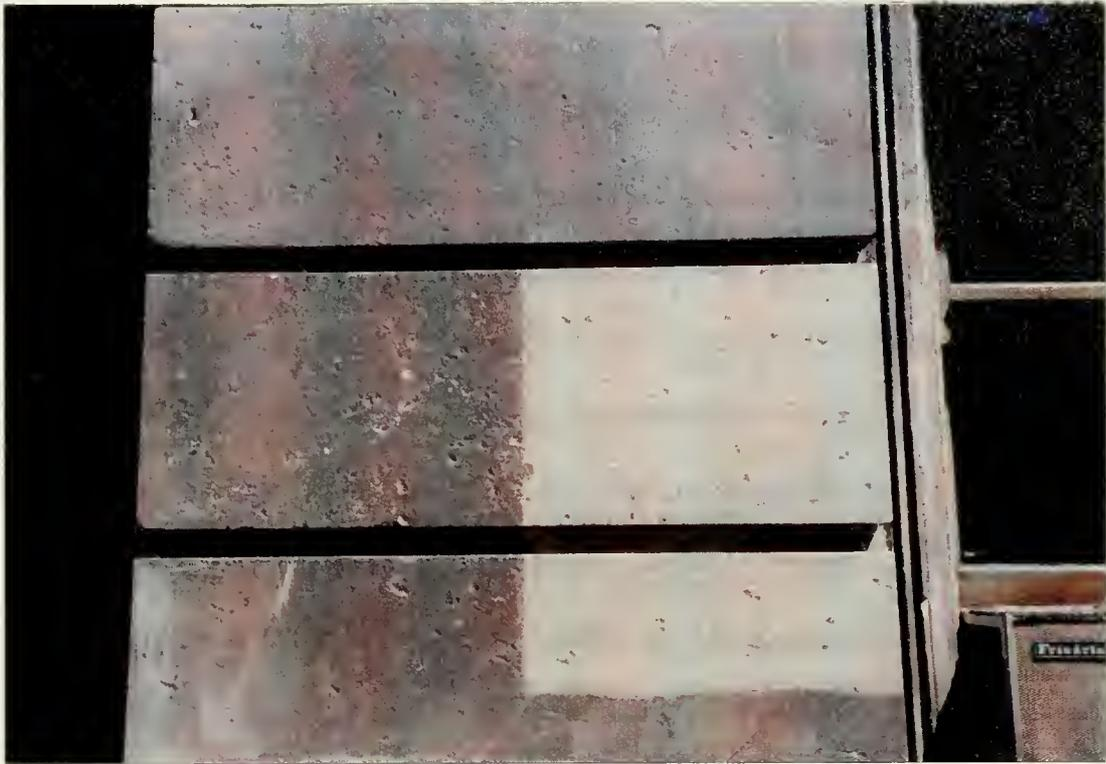
Figure 3.3: Cleaning test number 10 performed on two blocks of Tuckahoe marble at the first floor level, July 1989.
