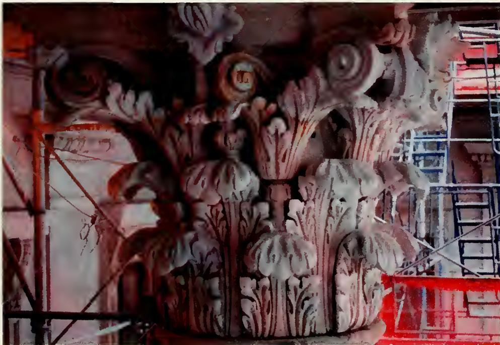
**Figure 5.2: Cherokee replacement abacuses on a Tuckahoe capital. Although the difference between the two types of marble is noticeable and will become more distinct as the stone weathers, the mixture of Cherokee with the Tuckahoe and Sheffield has been limited to areas of the building where it will not be as noticeable.**
