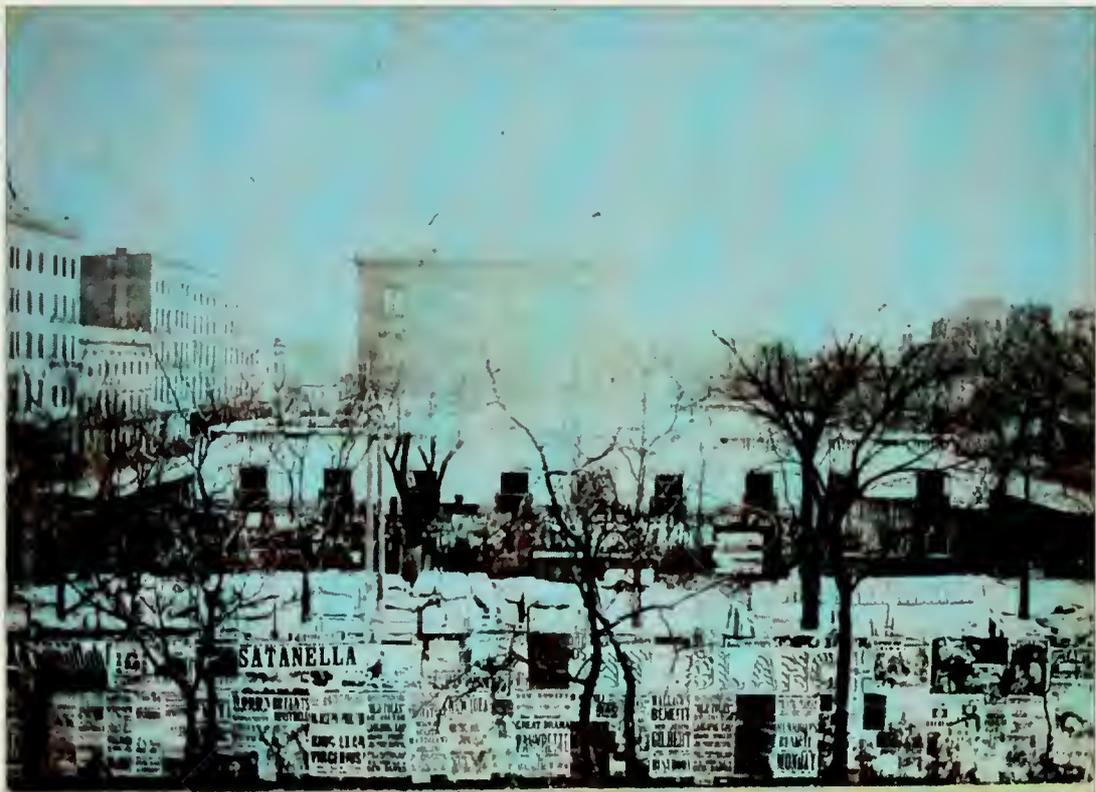
**Figure 2.2:** An 1863 daguerrotype of the construction site as seen from Broadway. Numerous blocks of marble lie in the yard directly behind the fence. A stonecarver's shanty appears to the right behind a line of carved elements, and a hoist is seen to the left of the image. Stonework has been completed on the first floor/ rusticated basement. Courtesy of the Scrapbook Collection, New York Public Library.
