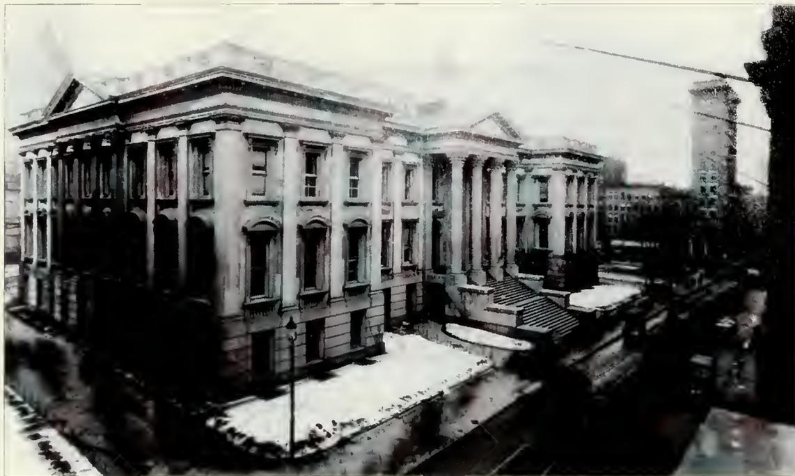
**Figure 2.4:** A circa 1900 photograph of the Tweed Courthouse as seen looking southwest across Chambers St. Discoloration of the juxtaposed Tuckahoe and Sheffield marble is evident even from this distance. The granite staircase to Chambers St. seen here was removed during the 40's. Photograph provided courtesy of John G. Waite and Associates.
