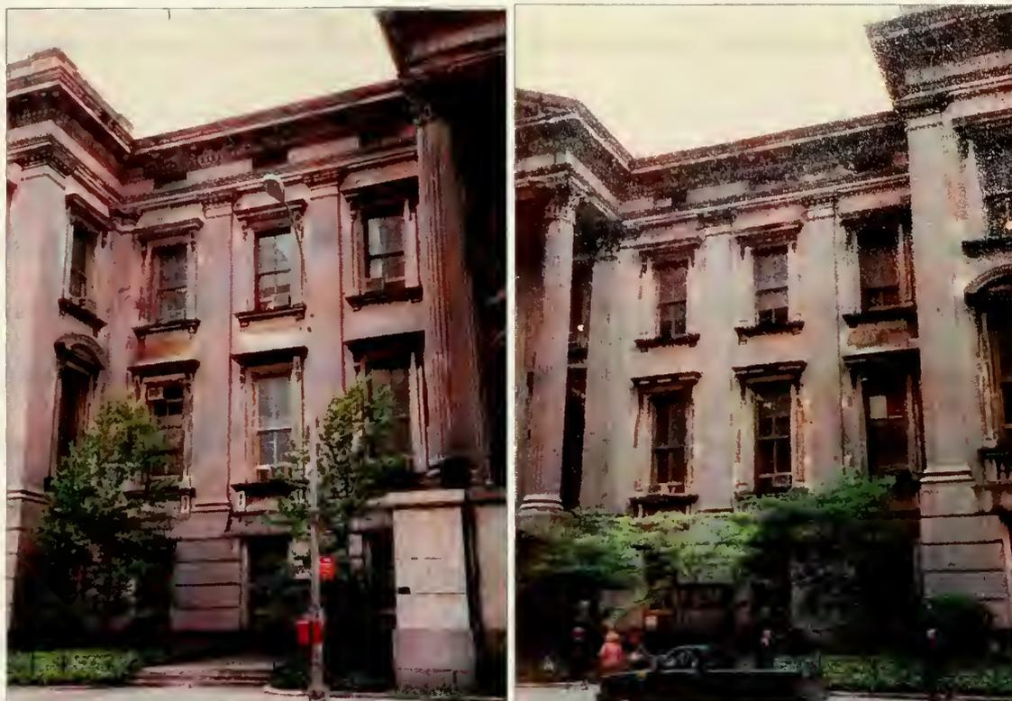
Figures 3.1 & 3.2: Discoloration on the north façade, east and west sides of the portico. May, 1989.
