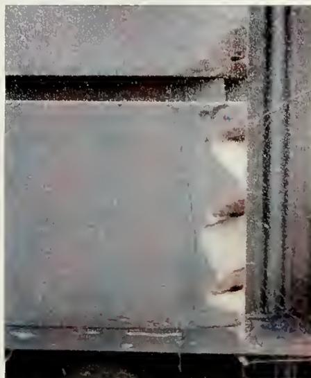
**Figures 3.6 & 3.7: Chipped pilaster flutes to the left and a chipped rusticated basement block to the right. Many of the finer details of the Tuckahoe marble have detached due to weathering. The whiter substrate has been exposed, revealing the level of discoloration. Photos taken May, 1989.**
