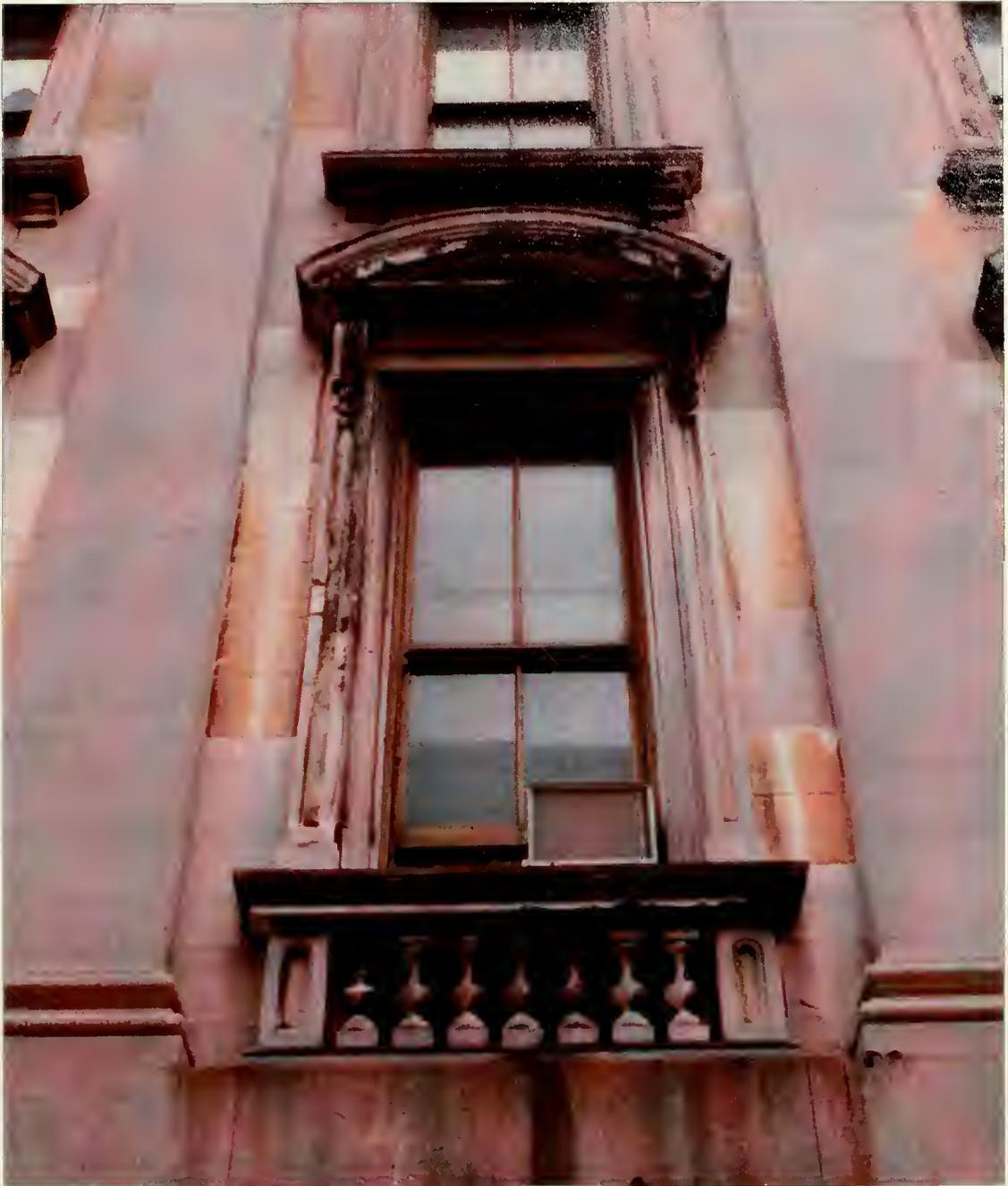
**Figure 3.16:** This photograph illustrates the juxtaposition of different stone types that is clear today but which was not obvious at the time of construction. Iron-stained blocks in the wall, probably Sheffield marble, are visually distinguishable from the gray, discolored stone, which is probably Tuckahoe. The window jambs both appear to be Tuckahoe, although the one on the left is significantly more chipped and discolored.
