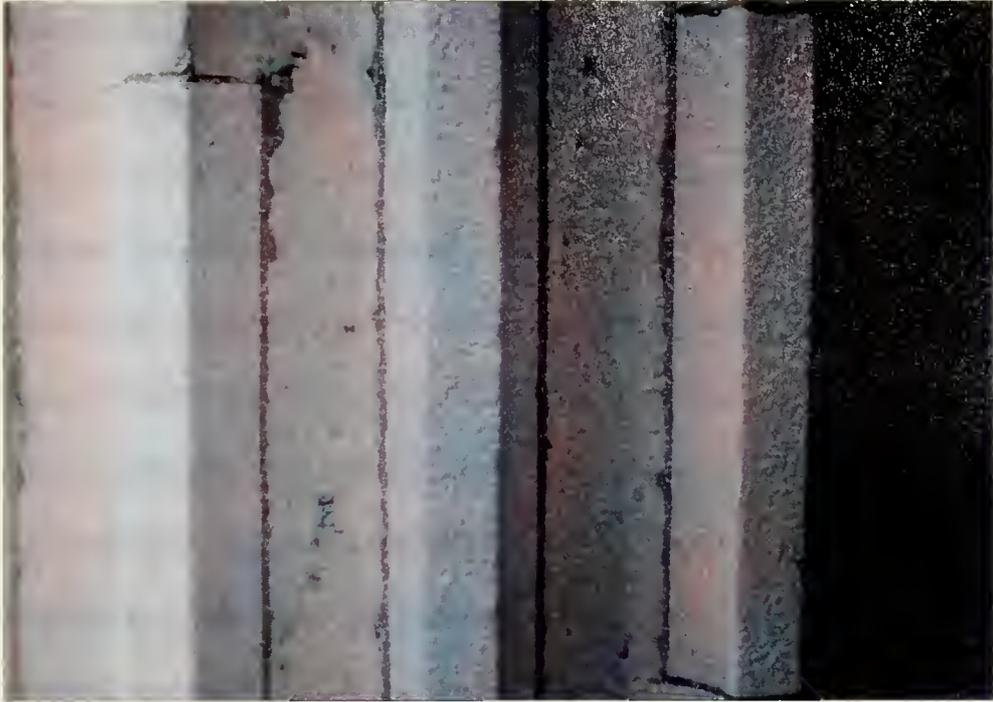
**Figure 5.1: Dutchman repairs to column flutes on Brooklyn City Hall. The one on the right is a closer match with the original Tuckahoe. After these repairs were made, extensive retooling was done to reduce the starkness of the contrast between the two types of marble.**
