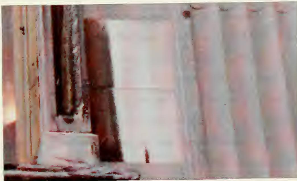
**Figure 3.14:** A combination of blackening and iron-staining on the left is non-existent on the right of these two blocks in the center of the photograph. The Similar to the iron-stained blocks, rain runoff appears to be washing part of the surface.
