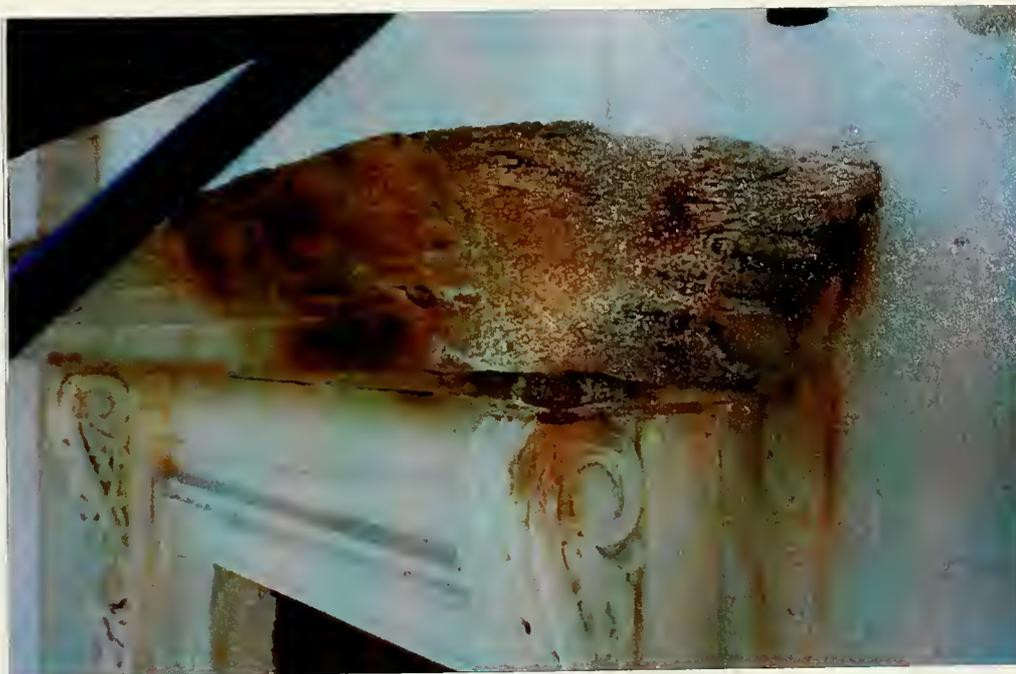
**Figure 3.13:** A Sheffield window header that had been covered with bituminous bird-proofing. The corner shows the effects of trapped moisture. This part of the stone could be removed merely by scraping the surface.
