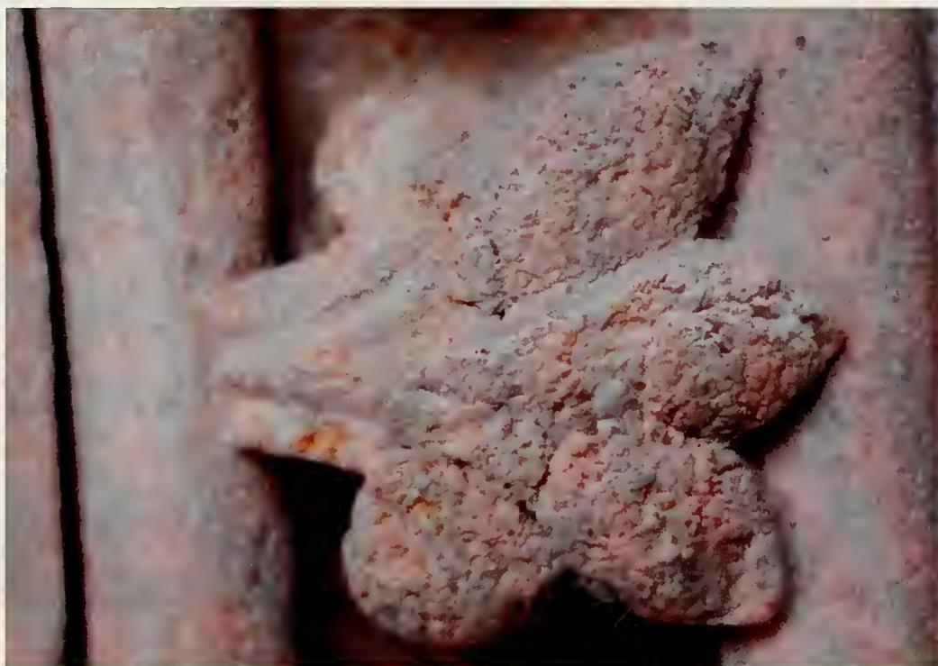
**Figure 3.8: Leaf detail with degraded surface showing exposed individual grains and iron stains. Weathering has made the surface extremely friable. Photo taken August 2000.**
