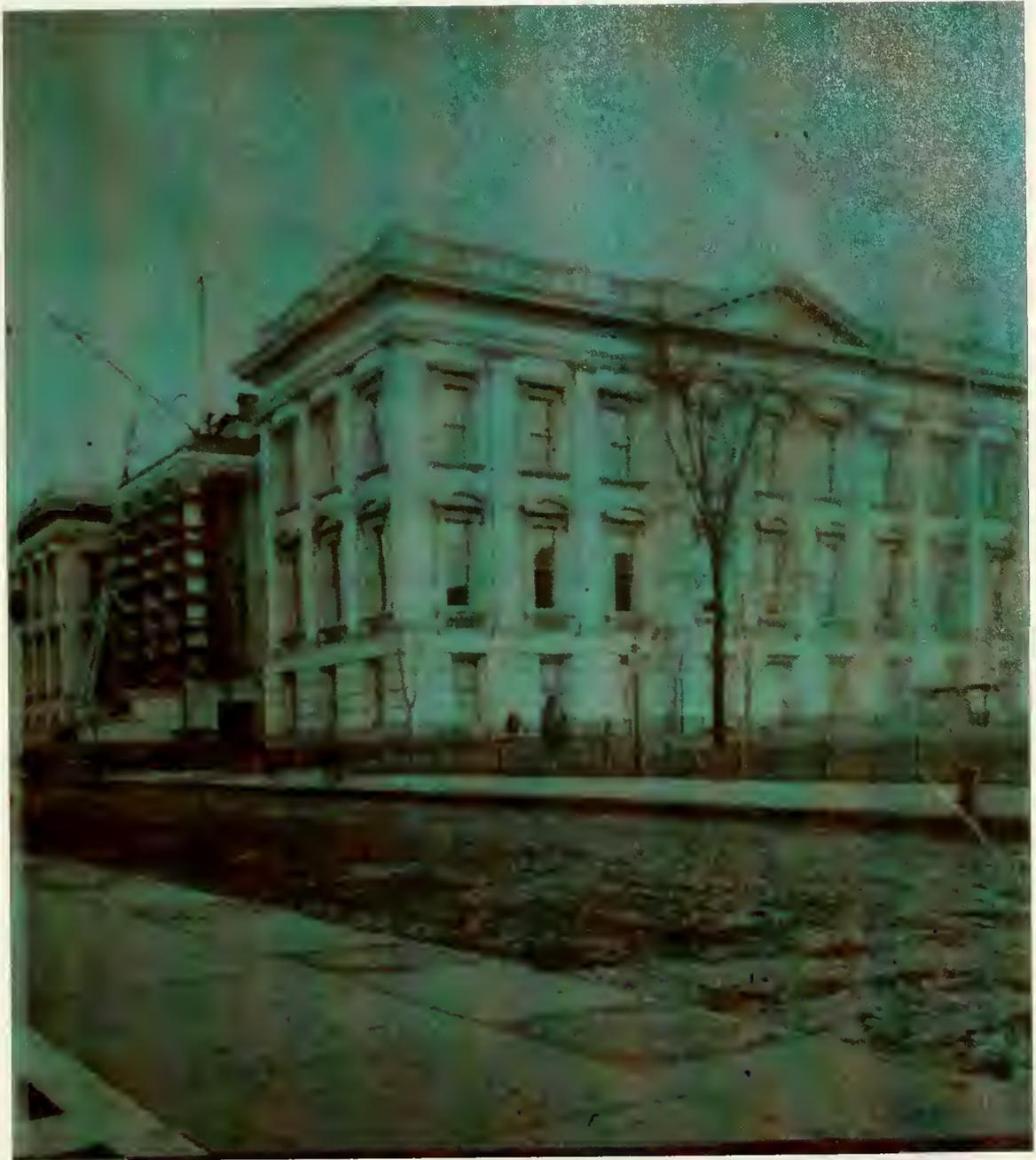
**Figure 2.3:** Image of the unfinished building taken from an 1873 stereoscopic photograph. The columns on the North Portico are not completed, and the pediment has yet to be installed. This view became emblematic of the plagued construction process. Courtesy of the Scrapbook Collection, New York Public Library.
