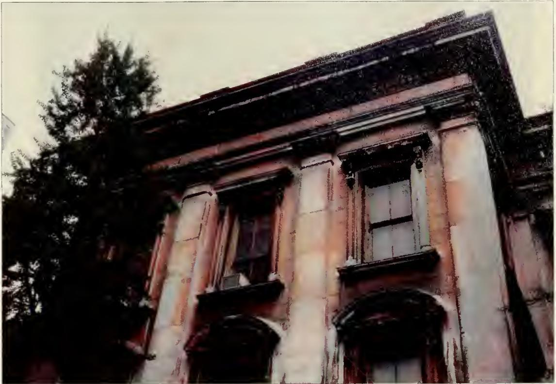
**Figure 3.11: South facade, west end, May, 1989. Extreme staining is visible across the entire surface. This type of discoloration is typical of Lee marble, a stone quarried within 20 miles of Sheffield, MA. The south façade exhibits the worst weathering on the building.**
