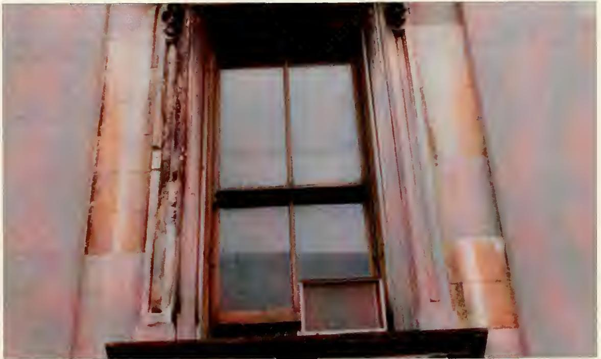
**Figure 3.10:** Iron-stained marble, probably Sheffield, interspersed with blocks of Tuckahoe. Iron staining may be due to the leaching out of ferruginous minerals such as pyrite. Note how the stone has been washed white in areas of rain runoff near the Tuckahoe marble while the Tuckahoe has remained a solid gray color. Photo taken May, 1989.
