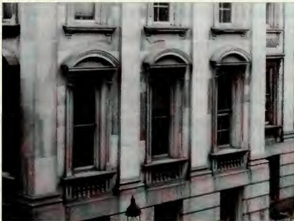
**Figure 2.5:** Close-up view of the same photograph showing differential staining of exterior marble around the second floor windows. The darker blocks are probably Sheffield marble.
