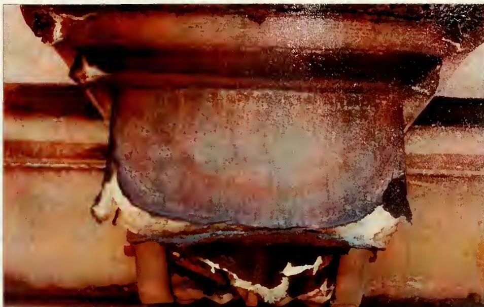
**Figure 3.17: A modillion appears to be splitting at the seams due to continued freeze/thaw cycling beneath a hard surface crust of gypsum. Note the semicircular patterns of brownish and blackish iron deposits due to the diffusion of iron leachates and other atmospheric pollutants.**
