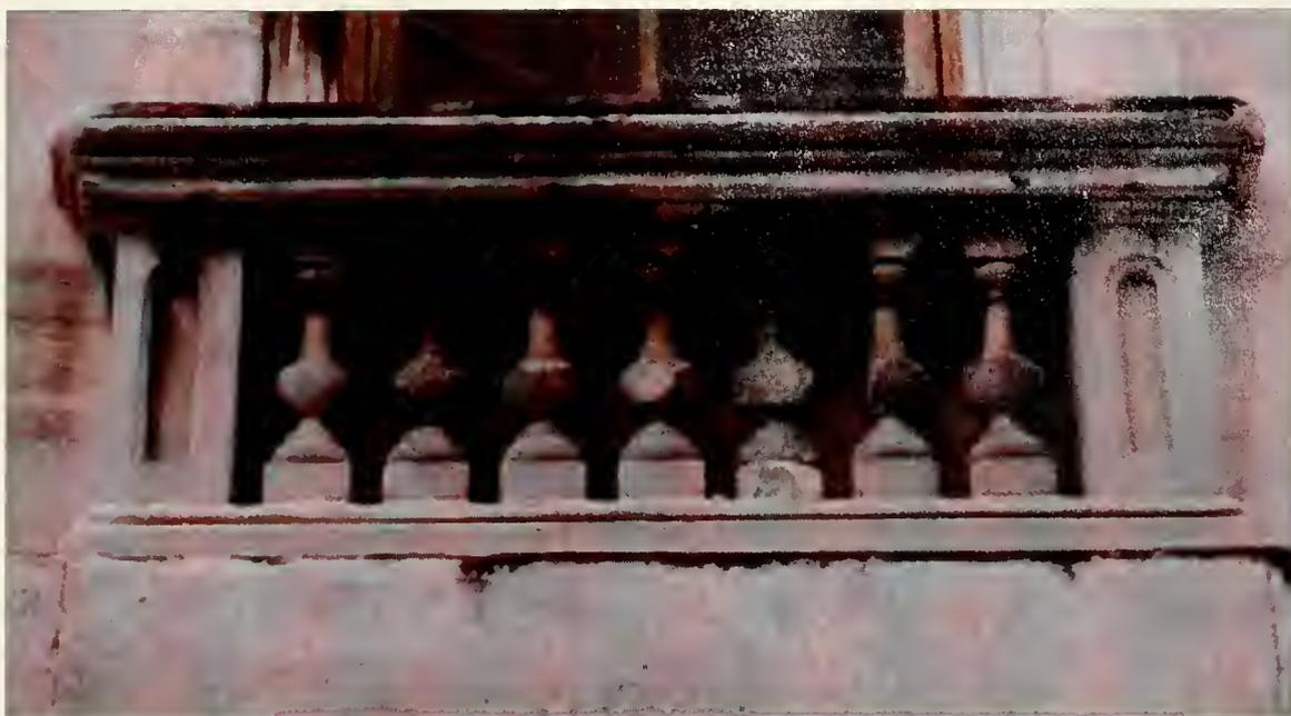
**Figure 3.5: Tuckahoe marble balusters showing extreme degradation due to weathering. Characteristic gray discoloration and blackening from the accretion of pollutants are evident. Projecting elements of both types of marble tend to look alike because of pollution staining. Photo taken May, 1989.**
