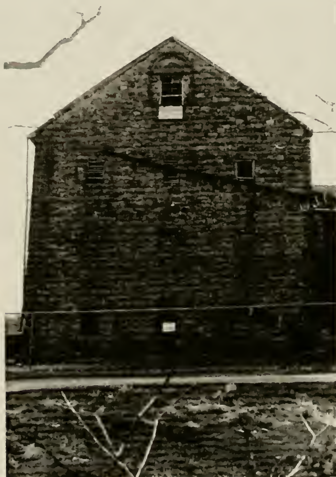
Plate 12: Close-up of east gable end showing symmetrical layout and recessed stone panels at middle level
