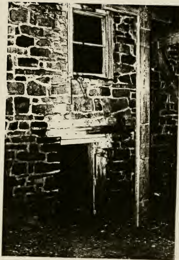
Plate 29: View of north elevation from carriageway in 1826 section, showing door leading into stables and window above into middle level, or granary
