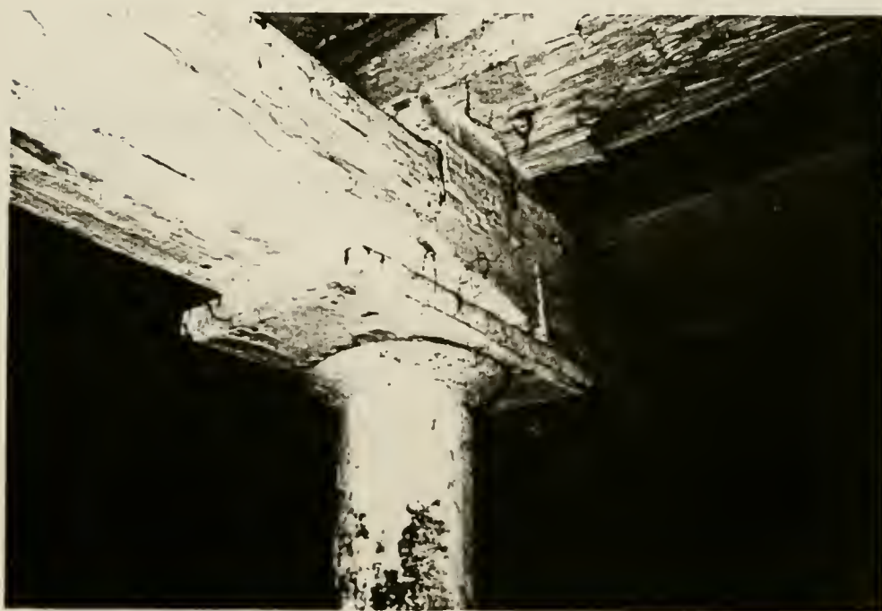
Plate 35: Detail of cast iron column and chamfered beam in 1826 stall section
