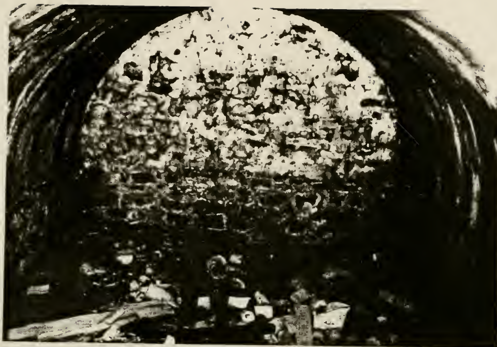
Plate 31: Stone vault #1 in 1826 ramp section, showing depth of room and whitewashed surfaces. This vault was accessed by an exterior door opening along southeast side of ramp retaining wall
