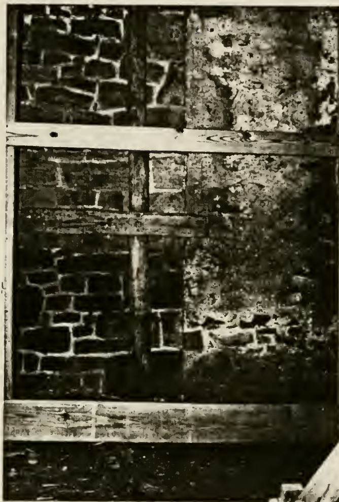
Plate 55: North elevation in carriageway section, showing exposed vertical seam between 1826 and 1845 sections. No attempt was made to disguise the joint on this elevation as opposed to south elevation.
