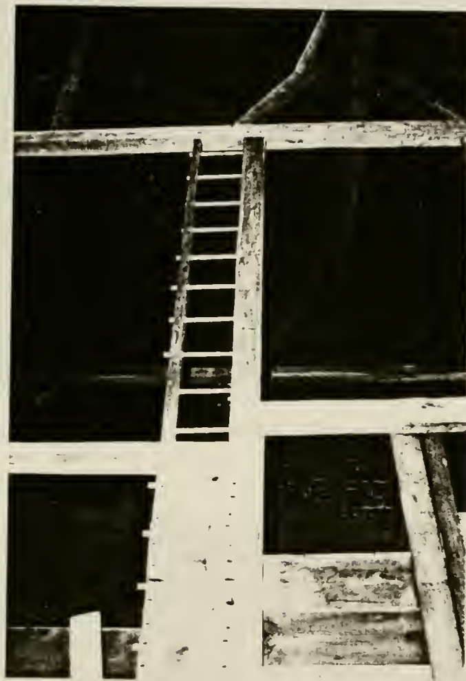
Plate 52: View west of 1826 structural framing, which employs a 3-bay H-bent design and system of diagonal braces at roof level. Note original west gable end in background.
