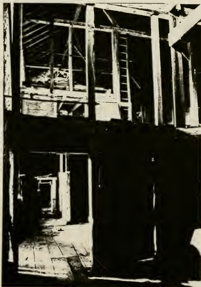
Plate 42: Middle and third floor levels of 1826 section, looking west, showing relationship of "sink-mow" and threshing platform
