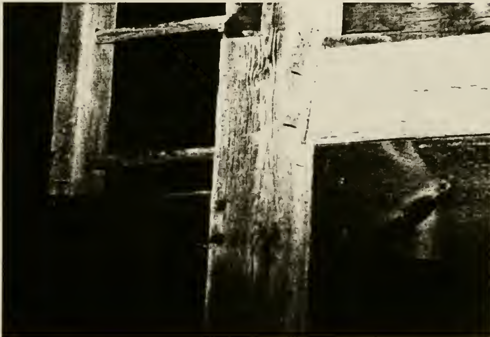
Plate 76: East side bent of 1845 threshing floor, showing detail of mortise-and-tenon joinery and numbering system on pieces.
