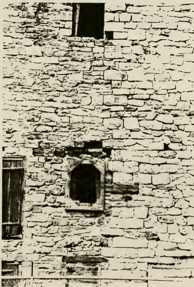
Plate 26: Detail of stone "dovetailing" on south elevation
