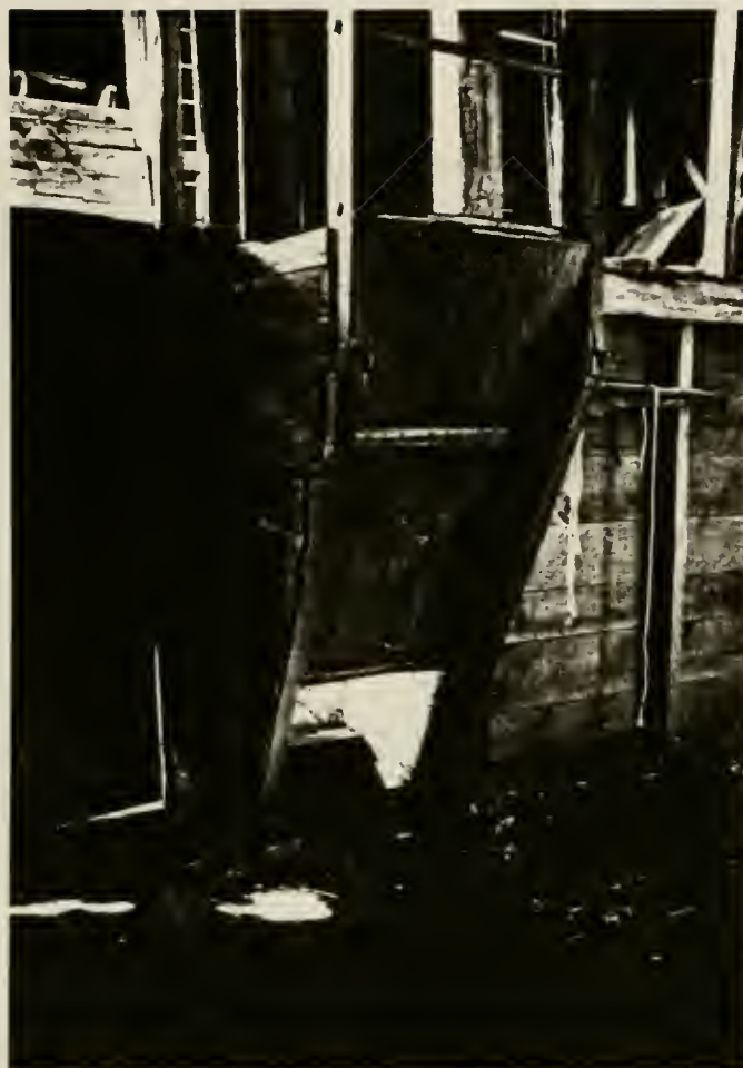
Plate 45: East hay mow of 1826 section, showing close-up of hay chute extending along side of threshing floor to floor below
