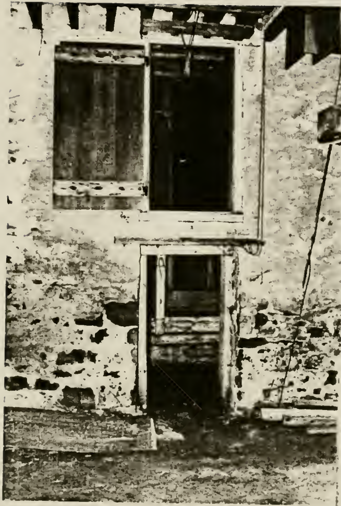
Plate 56: North elevation in carriageway of 1845 section, showing door into stables and door above to granary. Staircase along north wall of stall area provided access to upper levels. Note pieces attached to ceiling joists of barn bridge; location of machinery shown in Plate 57.
