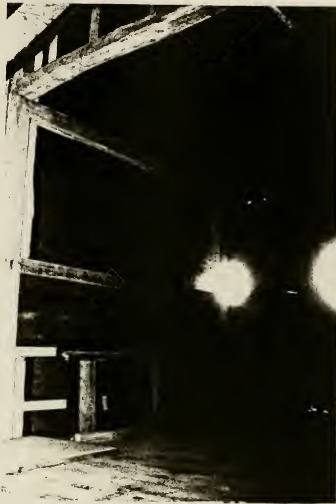
Plate 71: Threshing floor of 1845 section, looking southeast, showing typical H-bent, horizontal boards along lower part. Note "ventilator" poles in hay mow
