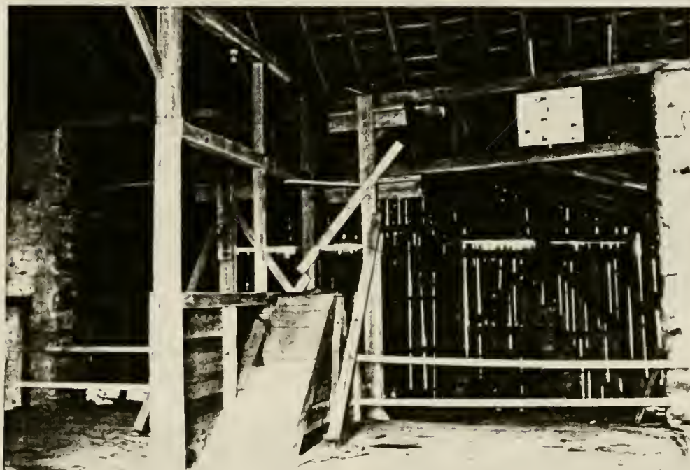
Plate 46: Threshing floor of 1826 section, looking north into rear shed addition. Two sets of double doors lead onto ramp. Note enclosed staircase (center) located in middle of platform. Pegs project from overhead cross beam above stair landing.
