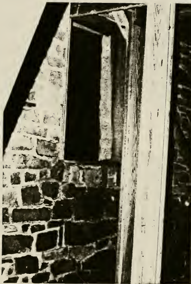
Plate 30: View of north elevation from carriageway in 1826 section, showing door to middle level, which was probably been reached by ladder. A staircase did exist along northeast end of stable area but has been covered over
