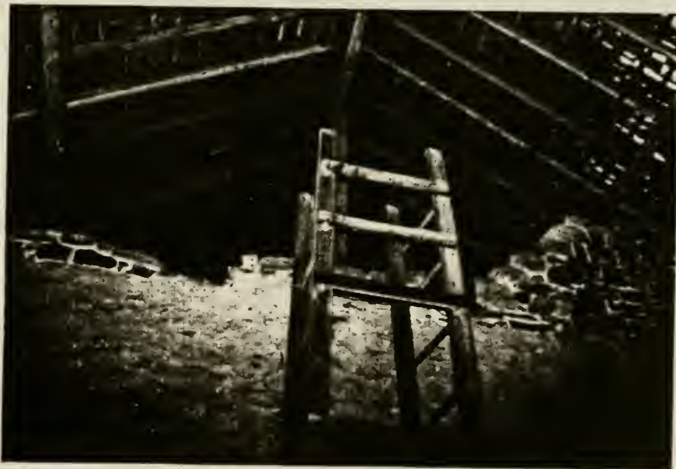
Plate 72: Close-up of ventilator poles. Note broken section of original west gable end
