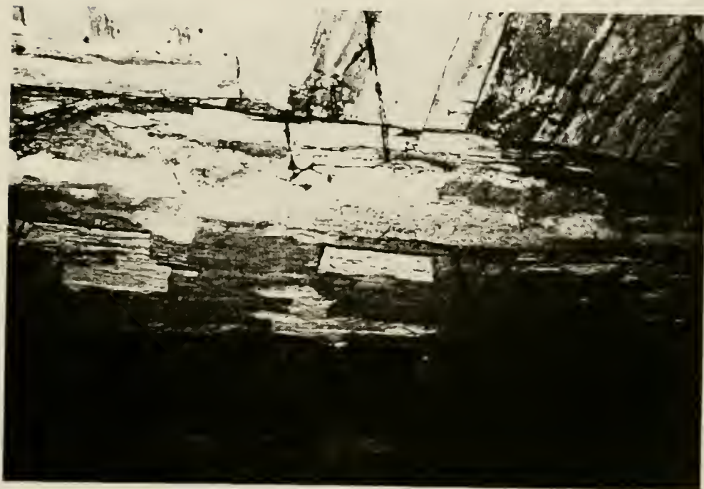
Plate 37: Detail of notches found in cross beam of 1826 stable ceiling framing. Holes may indicate location of earlier stall dividers (Refer to Appendix E for location of notches)
