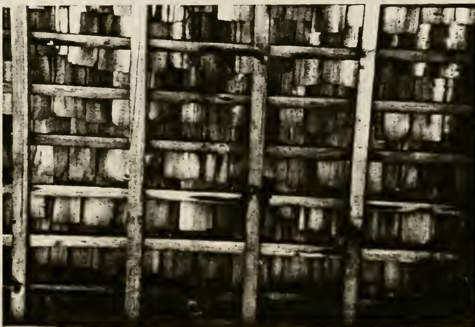
Plate 54: Close-up of 1826 roof above threshing platform, showing chain attached to framing which may have served as part of pulley system to unload hay wagons. Note shingled underside of roof.
