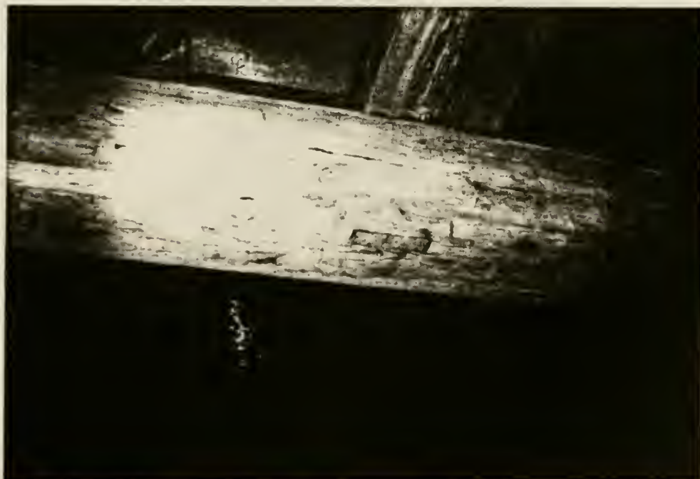
Plate 68: Detail of grain bin section showing evidence of cut diagonal brace along cross beam
