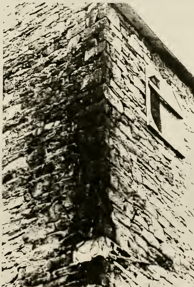
Plate 20: Detail of corner quoins along southwest edge of barn
