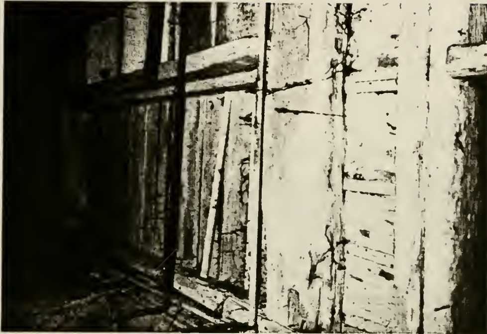
Plate 36: 1826 stall section showing evidence of closed staircase along northeast end, which would have led up to granary level
