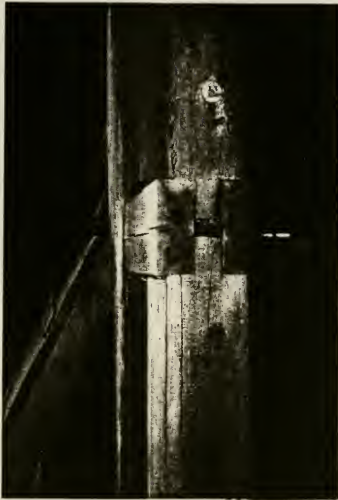
Plate 49: Detail of 1826 threshing floor framing, showing evidence of cut cross member
