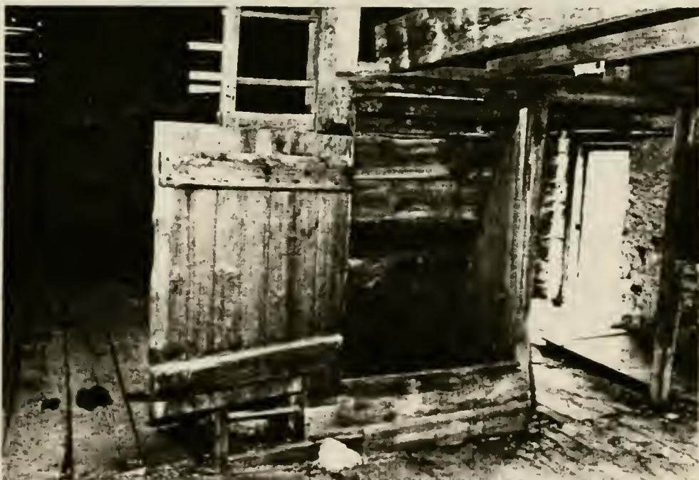
Plate 48: Threshing floor of 1826 section with view of hay chute opening, located along south side of platform. Note loft space above which covers part of south elevation.
