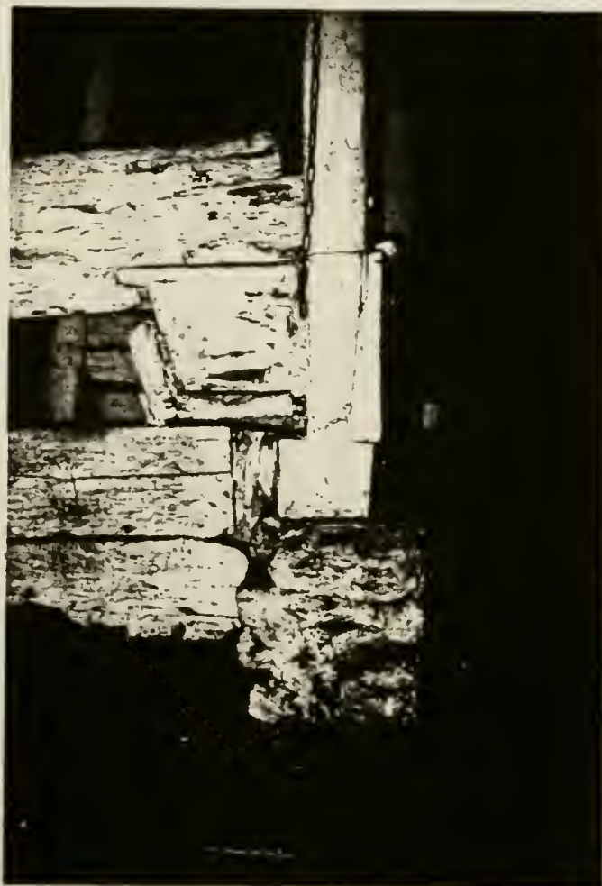
Plate 62: South stall area in 1845 section, showing broken stone foundation wall at midsection
