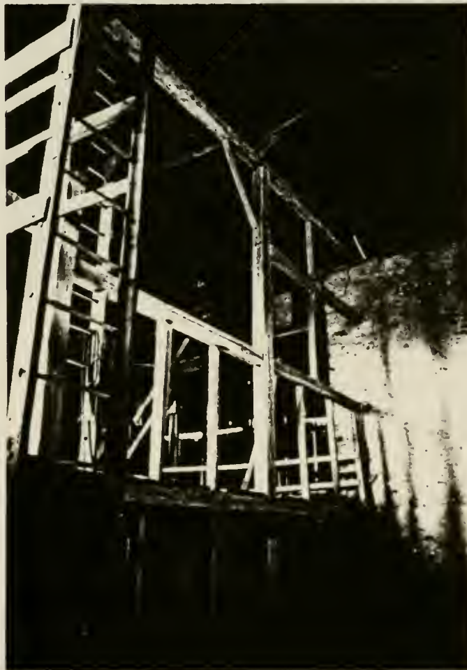
Plate 43: Threshing floor of 1826 section, looking east, showing window openings on east gable end and arrangement of typical framing (3-bay, "H-bent")
