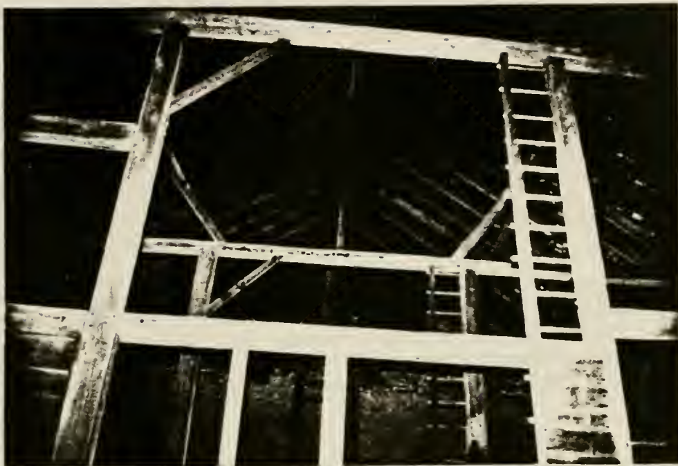
Plate 77: 1845 threshing floor, showing both bents located on sides of platform with view to original west gable wall. Note shingled underside of roof.
