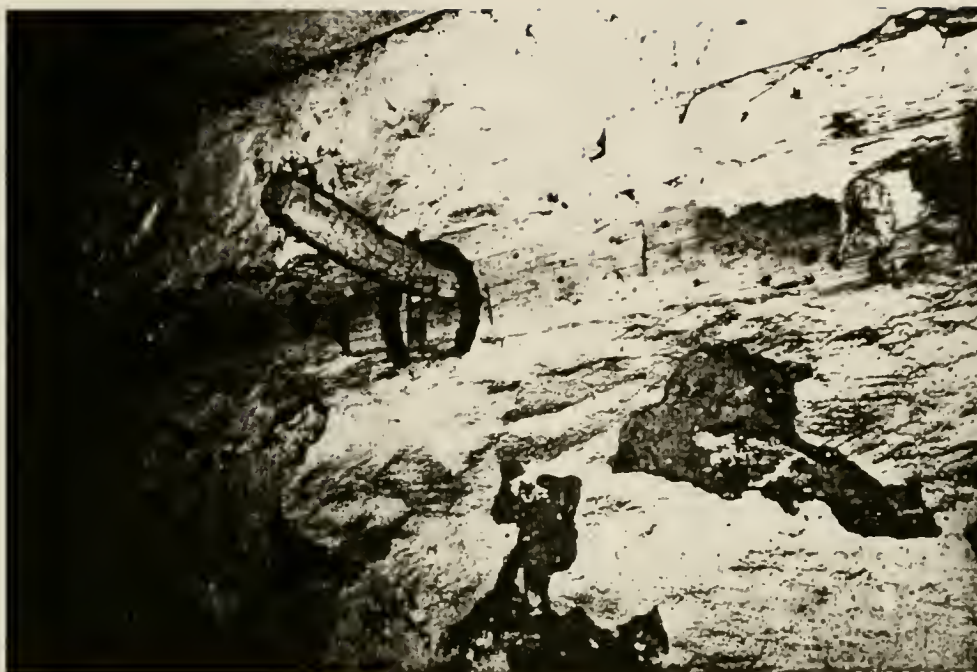
Plate 34: Pegboard embedded in east wall of 1826 stall section. Three pegboards are placed across the wall and would have been used to hang equipment
