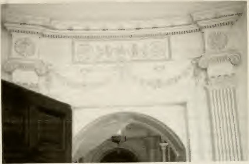
FIGURE 3.2.12 West door surround detail and door panel profile in the Oval Drawing Room. Photograph and drawing by author.
