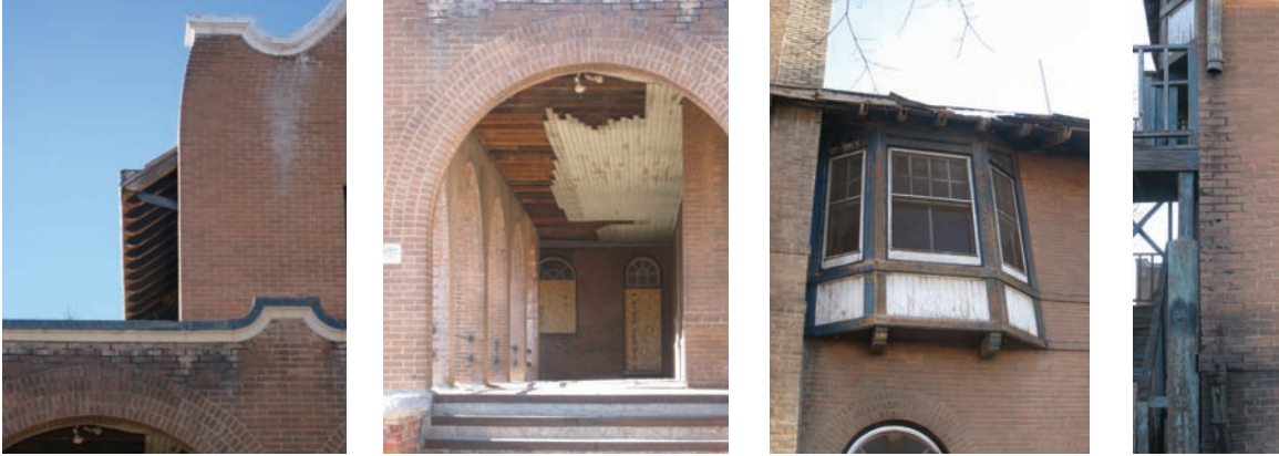
Figs 79-82 (l-r): La Castañeda currently suffers from mortar loss and roof drainage problems; threats to wood rafters; wood rot; and no gutter connections to move water away from the foundations.
